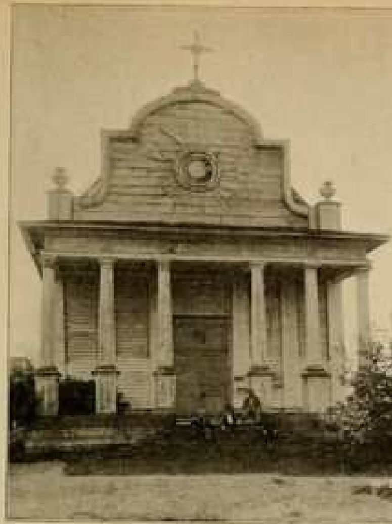
OLD MISSION AT CATALDO, KOOTENAI COUNTY. BUILT IN 1844. NO NAILS USED IN ITS CONSTRUCTION
